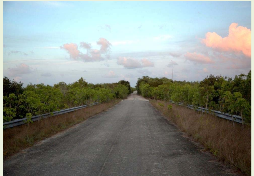
424 th Street, South of Florida City, East of US1
